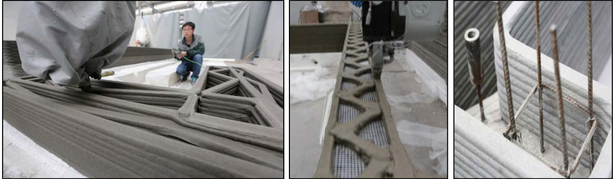
Figure A.21 – Yingchuang printing process including reinforcement (Yingchuang, 2015)
